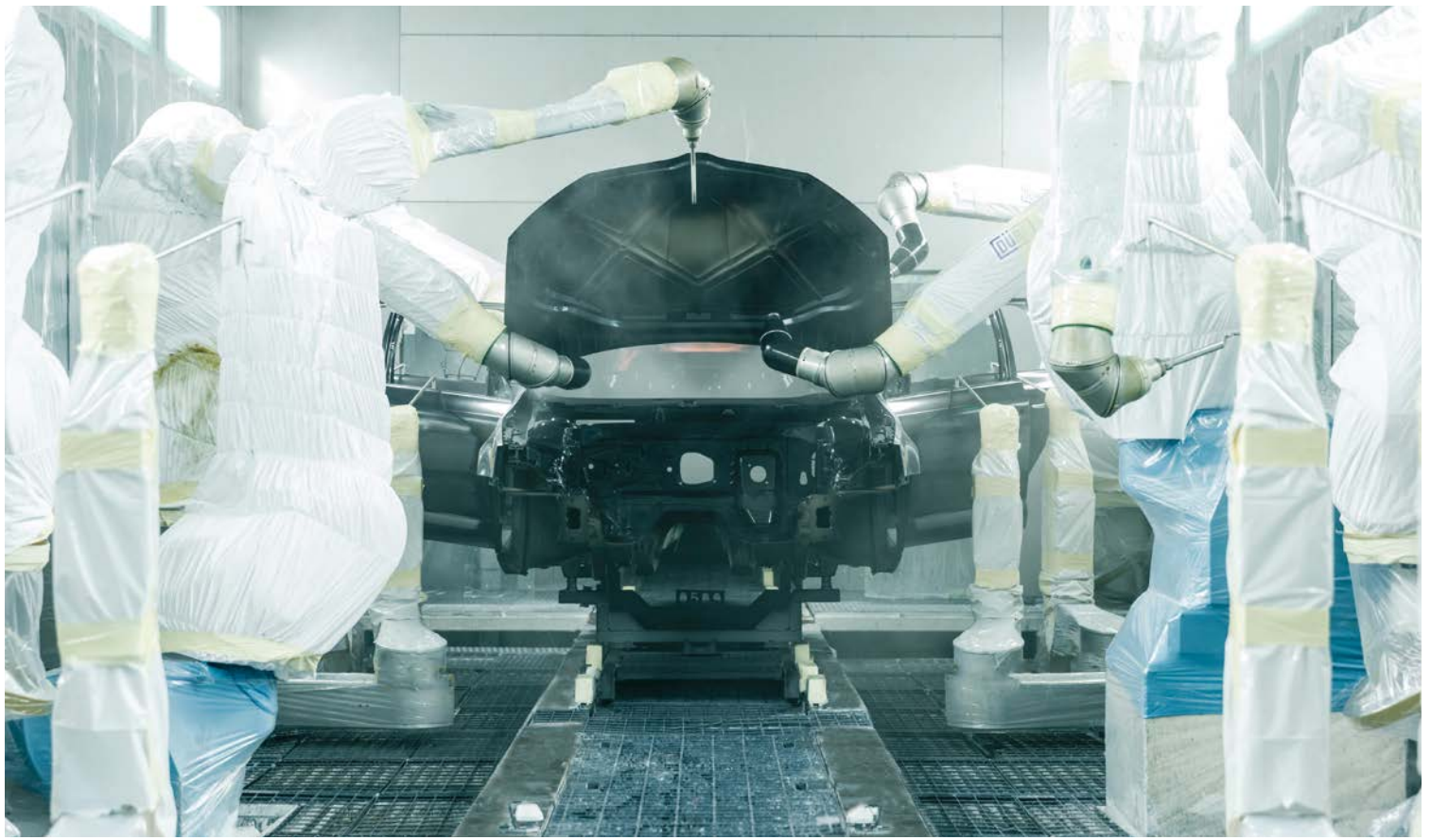
To improve product quality and increase system availability, the paint shop uses BSR's APROL ConMon solution for online vibration diagnostics.
