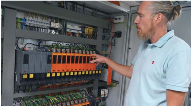
The open Ethernet-based real-time POWERLINK bus connects the entire production line to the heart of its control system.
